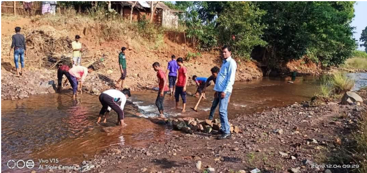
TEMPORARY WATER STAGNATION FOR VILLAGERS
